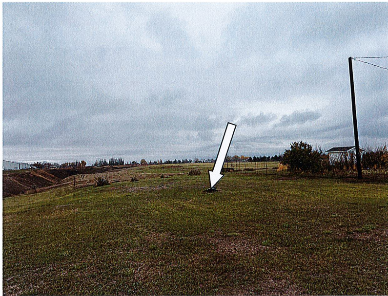
Photograph 2 – Looking east along north property line. Note catch basin Previously installed in preparation for storm sewer connection (arrowed)
