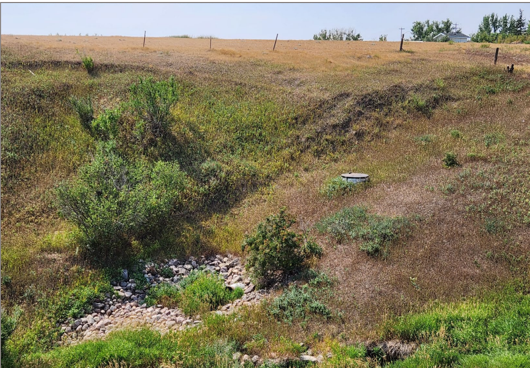
Photo 6: Culvert Along Site Slope.
